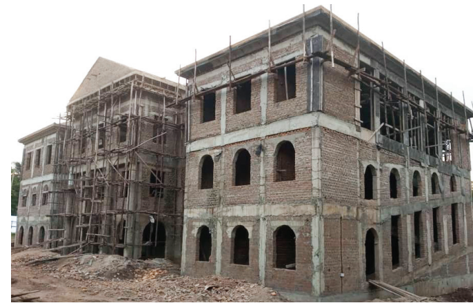
Above, Tororo High Court construction
