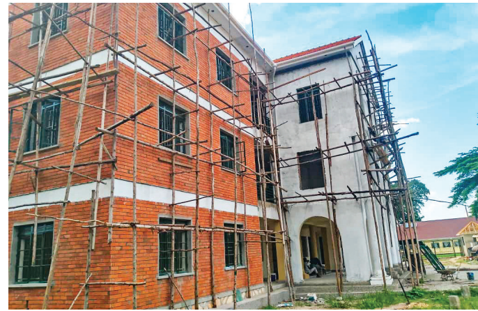
Soroti High Court Building
